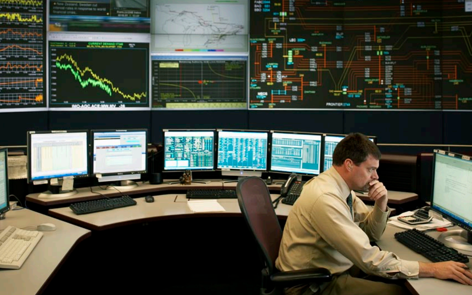
IESO Control Room
