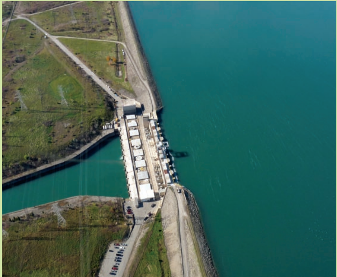
The Sir Adam Beck Pump Generating Station in Niagara provides 174 MW of electricity by using excess generation capacity to pump water from the Niagara River into a 300 hectare reservoir.
