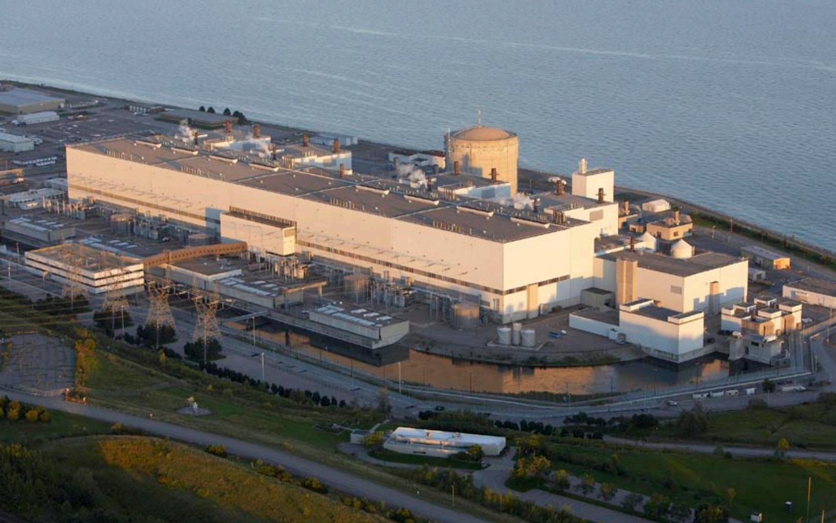
Darlington Generating Station
