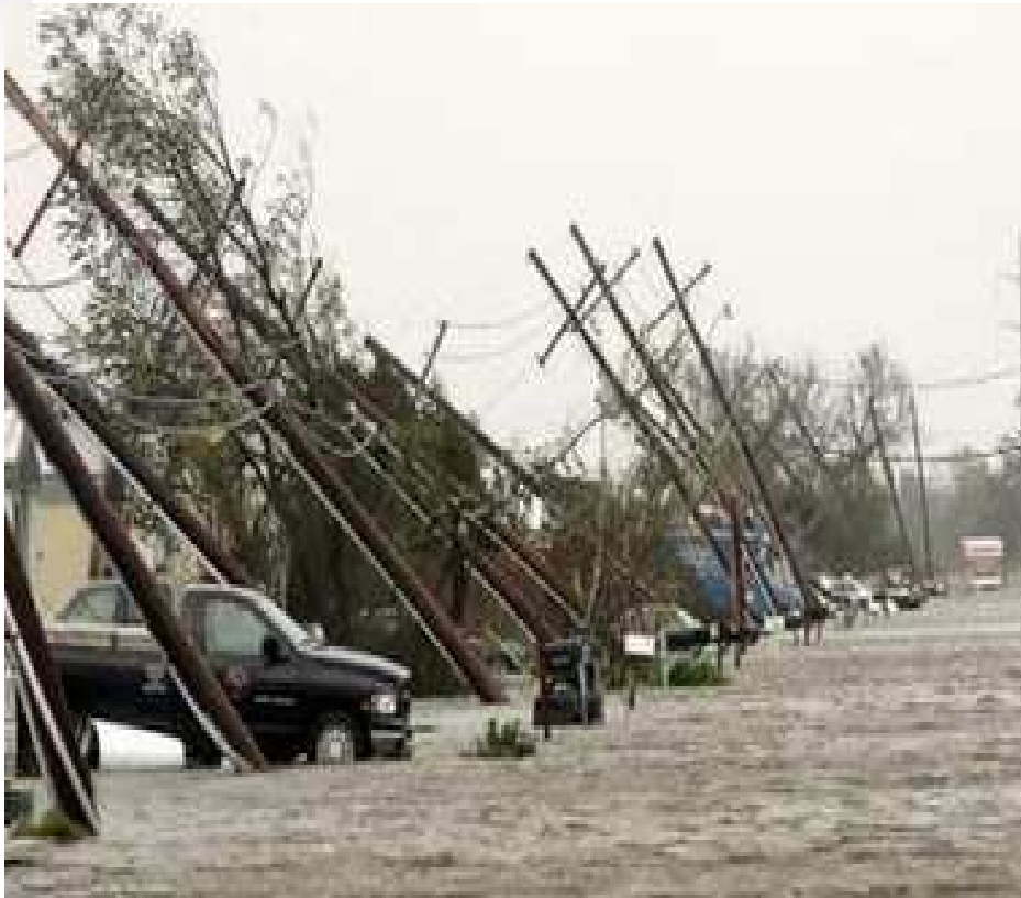
August 29, 2005: Power poles are pushed over in a flooded street after Hurricane Katrina
