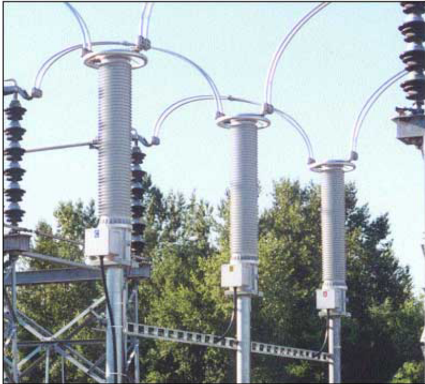
BC Hydro's Ingledow Substation – 230 kV Combined Voltage & Current Optical Sensor
