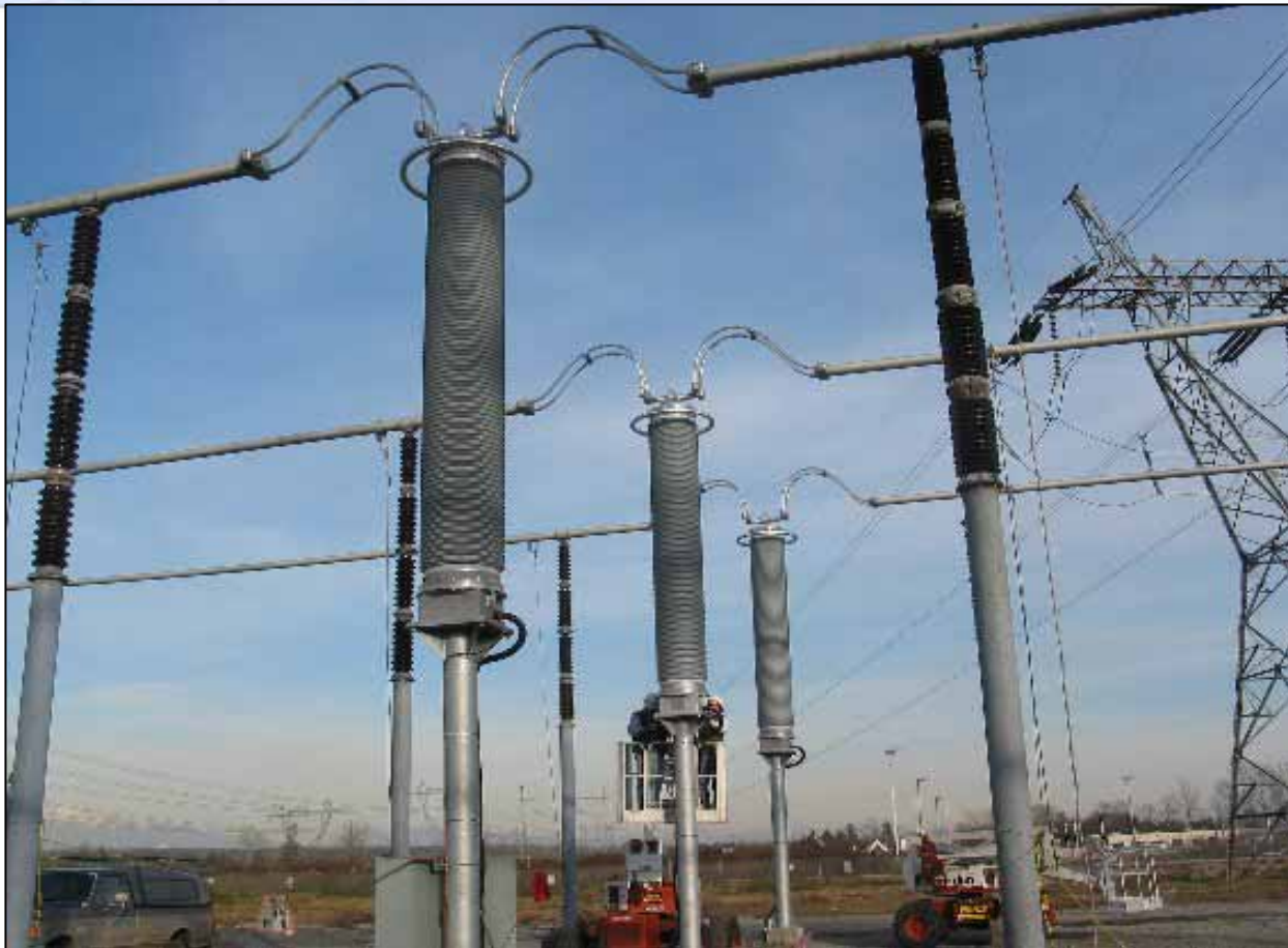
BC Hydro's Ingledow Substation – 500 kV Combined Voltage & Current Optical Sensor
