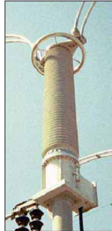
BC Hydro's Ingledow Substation – 230 kV Combined Voltage & Current Optical Sensor
