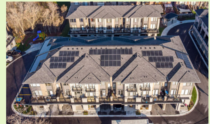
An increasing number of electricity resources such as small-scale solar generation are connecting directly to the local distribution grid. Engaged consumers and communities investing in these local resources are leading to a more diverse and decentralized system.
