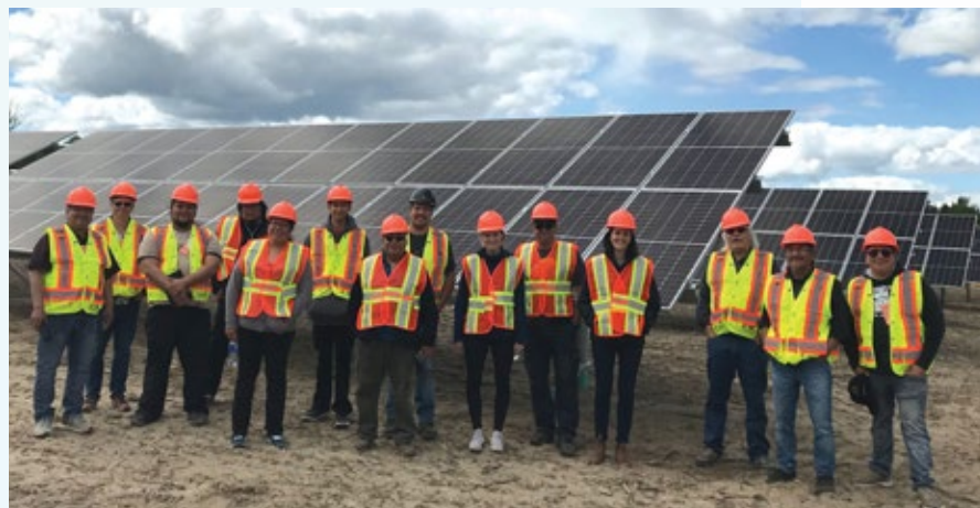
While in Kiashe Zaaging Anishinaabek – Gull Bay First Nation, CEC trainees had a chance to visit the community’s microgrid project, which combines solar power, battery storage and smart grid technologies.
