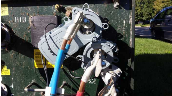
Distribution transformer monitoring equipment Image source: Grid 20/20 and Ontario Ministry of Energy
